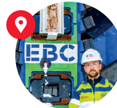
PIERRE CR116 – Ang Mo Kio Station & Tunnels
