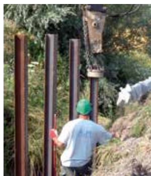
Battage des supports
