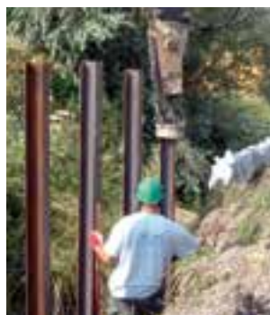
Battage des supports
