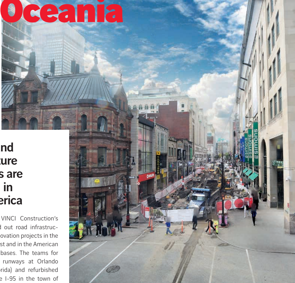
Renovation of Sainte Catherine street in Montréal (Québec), Canada.
